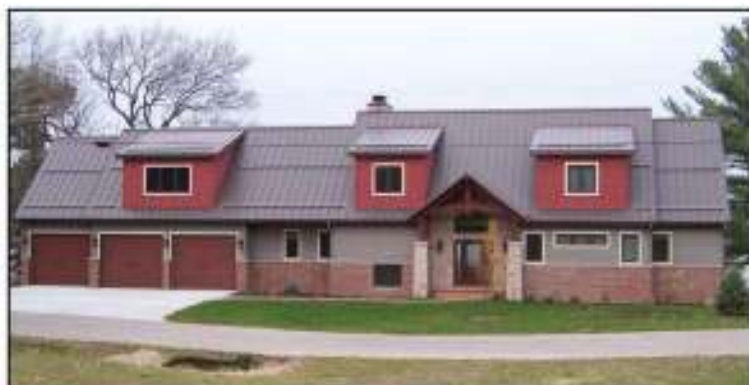
Metal Roofing: 5,957 sqft. - 2009124200
