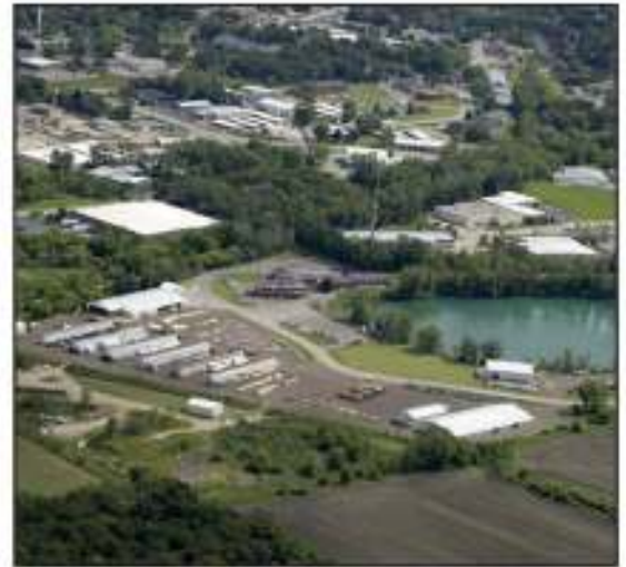
World Headquarters and Flagship Manufacturing Plant Verona, WI
