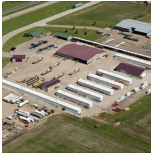
Midwest Manufacturing Plant Grand Island, NE
