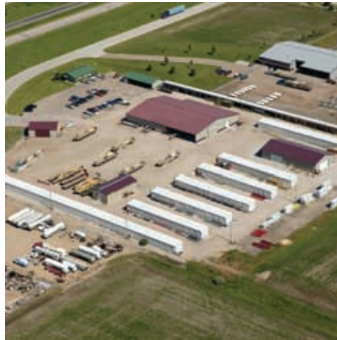
Midwest Manufacturing Plant Grand Island, NE
