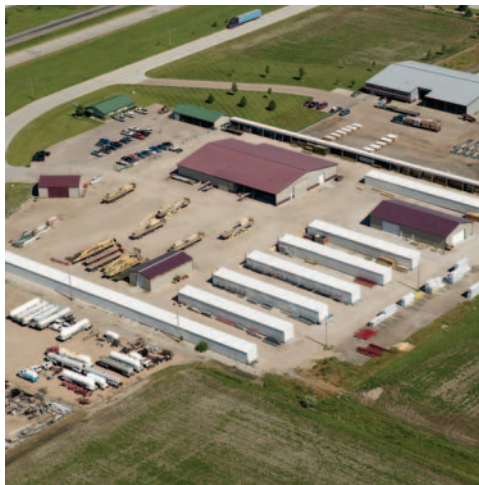
Midwest Manufacturing Plant Grand Island, NE
