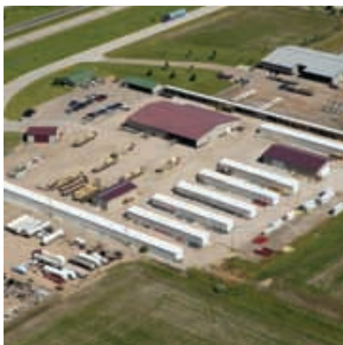
Midwest Manufacturing Plant Grand Island, NE
