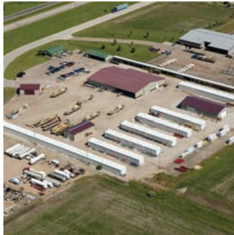
Midwest Manufacturing Plant Grand Island, NE
